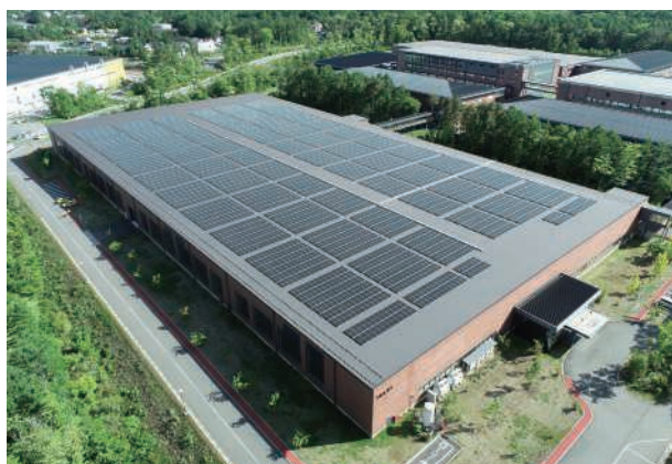
FANUC Headquarters (Reliability Evaluation Building)
