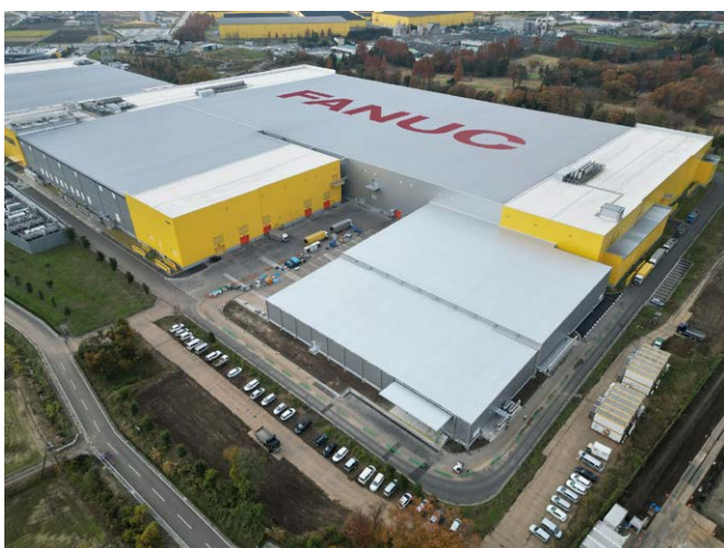
Tsukuba Robot Factory #1/Finished products warehouse
