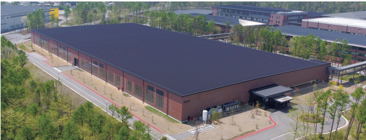
Reliability Evaluation Building
