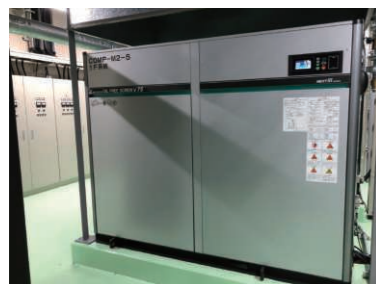
3 Energy-saving compressors (inverter type)
