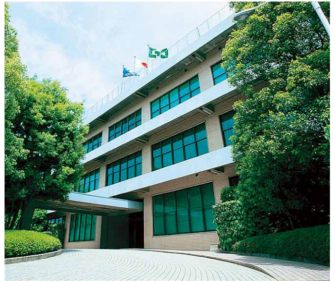
Kariya head office factory
