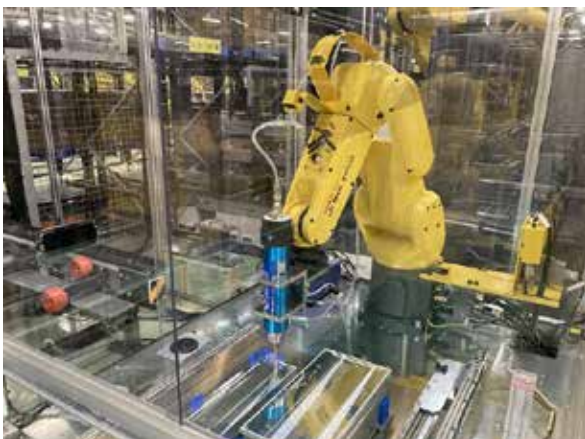
Robot module applying sealant
